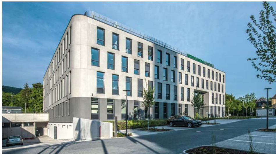
Heidelberg Technology Center (HTC) in Leimen, Germany: one of its main research topics is the reduction of CO 2 emissions.
